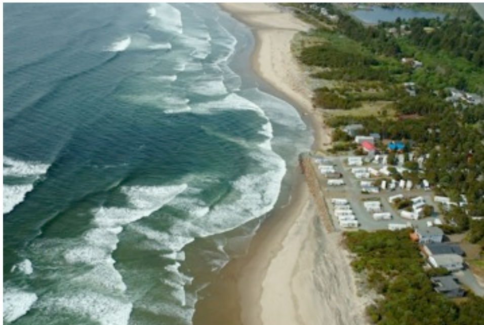
Figure 9. Ongoing shoreline retreat over the past decade in the Rockaway cell and localized hotspot erosion effects have resulted in substantial sections of the shore having to be rip-rapped in order to safeguard property. SLR expected over the next century and enhanced storms will almost certainly increase the risk of failure of such structures and the potential loss of homes and important infrastructure backing the beach (Photo courtesy of Mr. Don Best, 2009).
